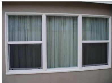
New vinyl windows set between existing wood mullions
